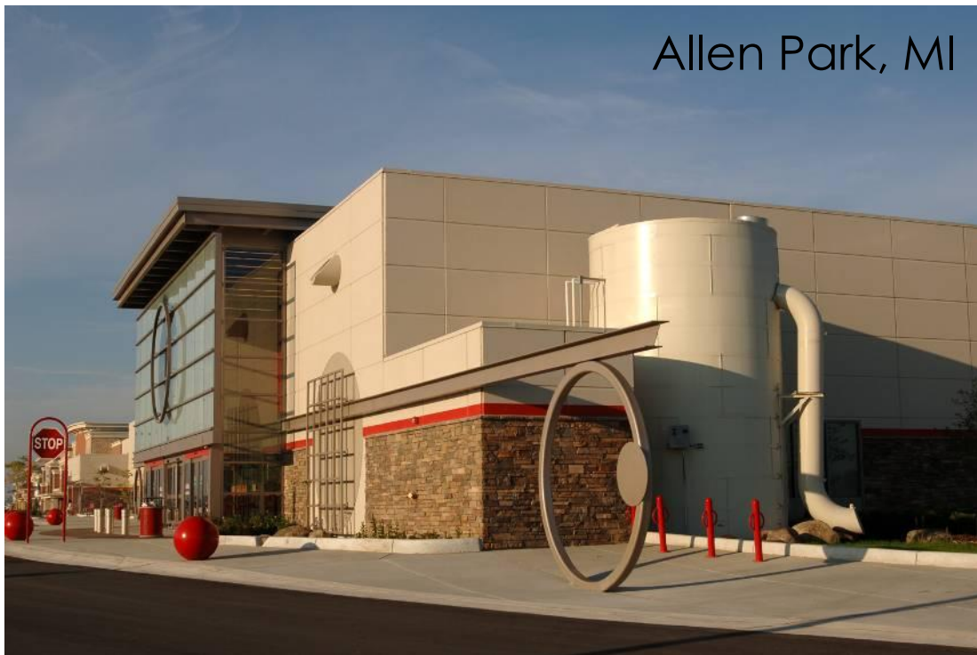
Rainwater capture storage tank
